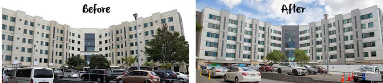
Scott Building cladding remediation work (before and after pictures)
