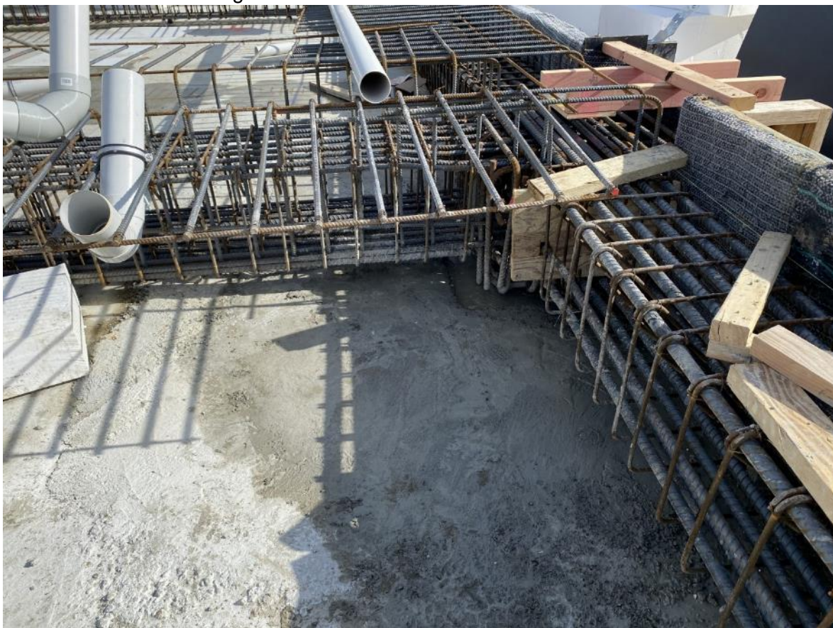
Ground beams reinforcing
