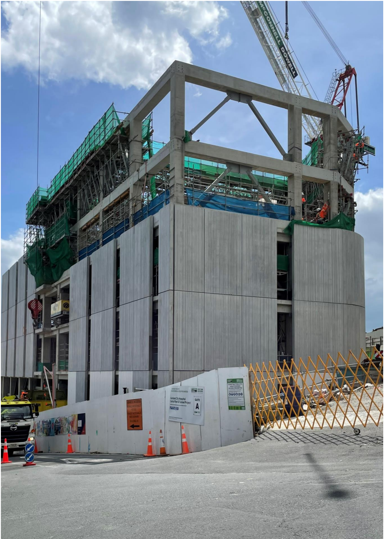
Building A40 – Facilities Infrastructure Remediation Programme Tranche 2, Auckland
